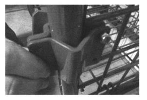
Step 2: Install the three 1/4-20" by 1" bolts to bracket and install 1/4-20" nuts as shown in the photo below.
