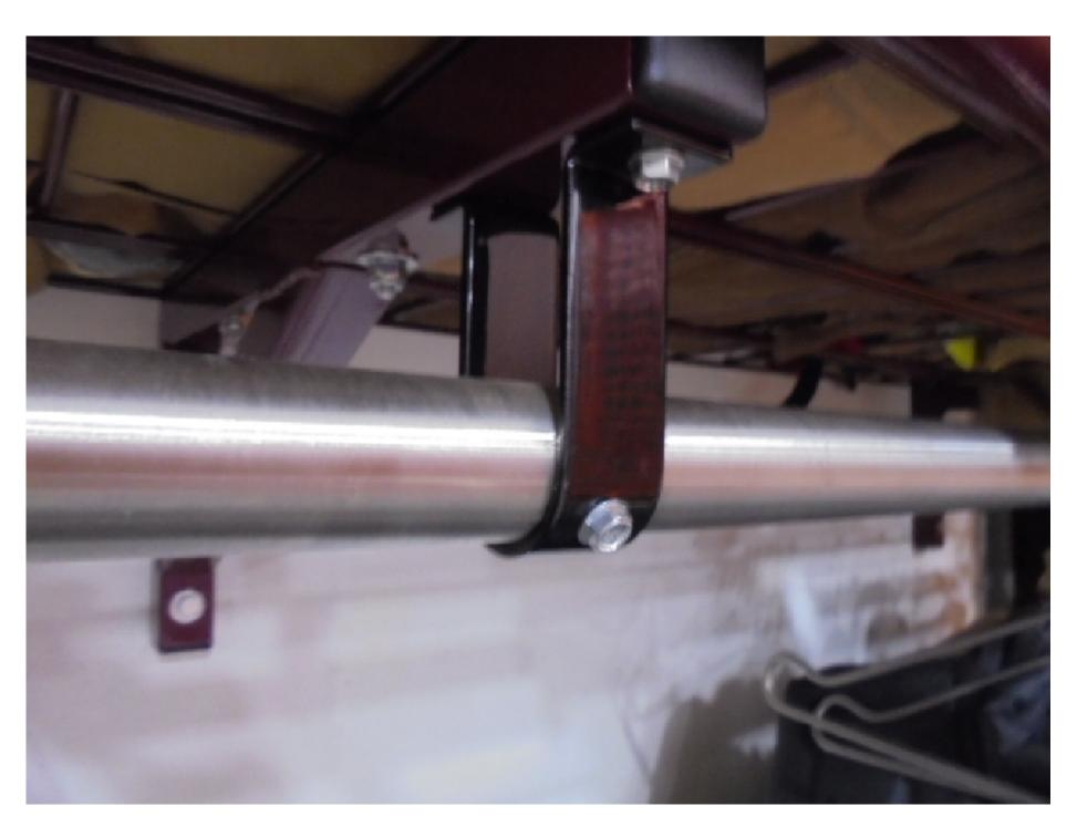
**STEP 5 (OPTIONAL HANGBAR):** PLACE HANGBAR IN HANGBAR BRACKETS AND USE THE SELF DRILLING SCREWS TO MOUNT TO THE SHELF BRACKETS.
