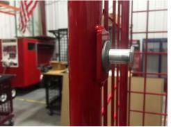
Step 7. Attaching door latch assembly per door. Place door latch to door as shown in the picture. Use two ½-20 x ¾" fasteners and install to the bottom two holes as shown. Next install the thumb latch and the washer, position washer between the door latch and the thumb latch as shown in the image. Use the last ½-20 x ¾" fastener to secure the thumb latch (do not over tighten this fastener as it could cause the thumb latch to not move)
