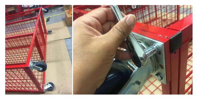
Step 6. Grab top, and insert (8) 5-1/2" bolts, washers, and wedge nuts. Wedge nuts must be in this orientation. (See photo)
